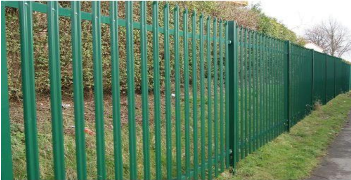
Image 4.14: Steel Palisade Fence
