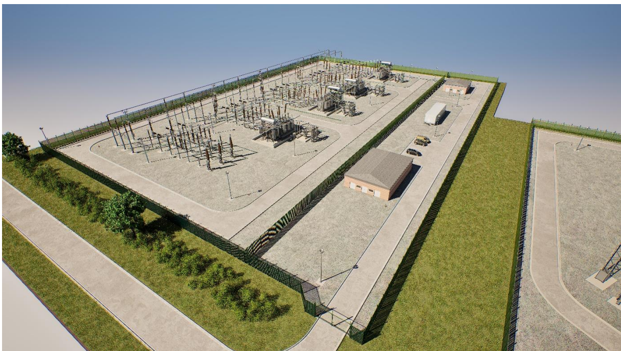
Image 4.10: Air Insulated Substation
