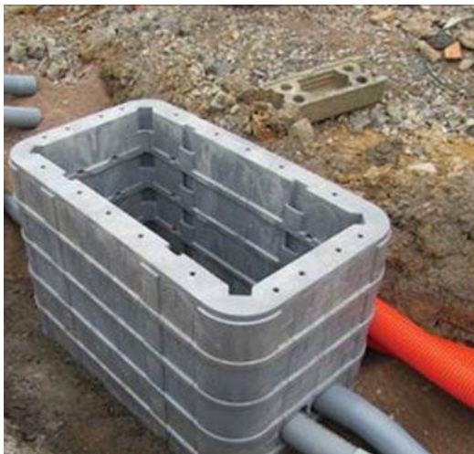
Image 4.12: Fibre Chambers (Construction and External Appearance)
